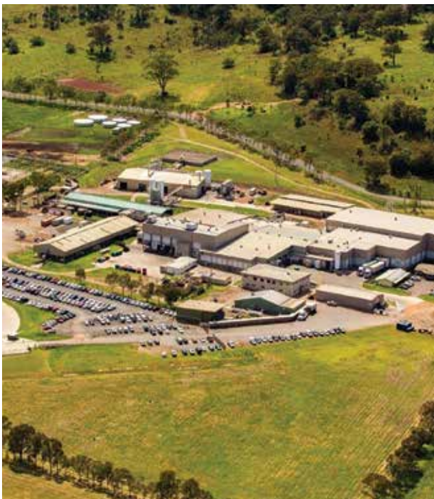
Aerial view of the JBS processing plant
